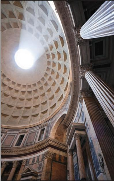
Completed in 125 AD, the enduring Pantheon, and in particular, the dome, was constructed with pumice aggregate and pumice pozzolan-enhanced concrete. Almost 2000 years later, the Pantheon is still the world's largest unreinforced concrete dome.
